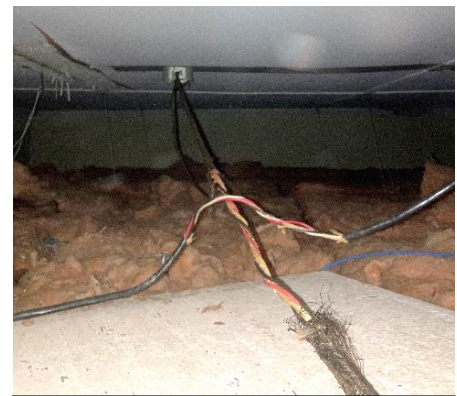
Bare wiring in the Parish Hall ceiling
